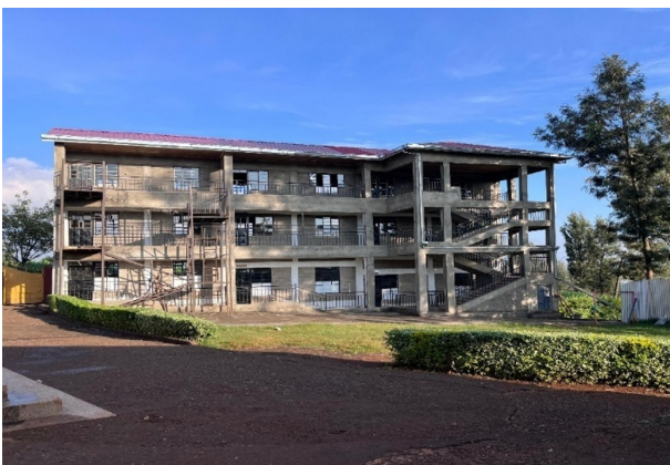
Sifa House under construction.
