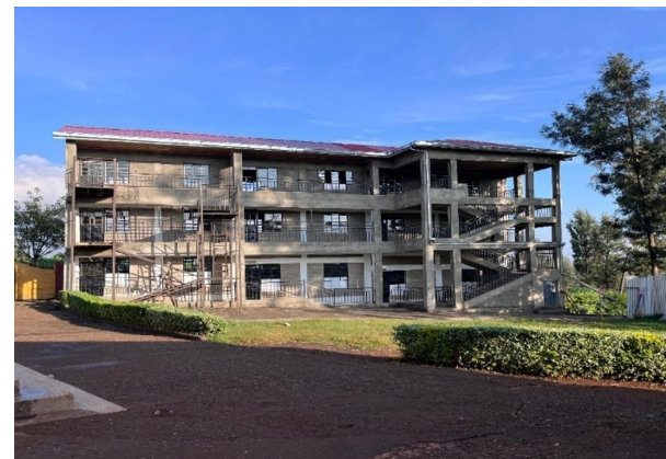
Sifa House under construction.
